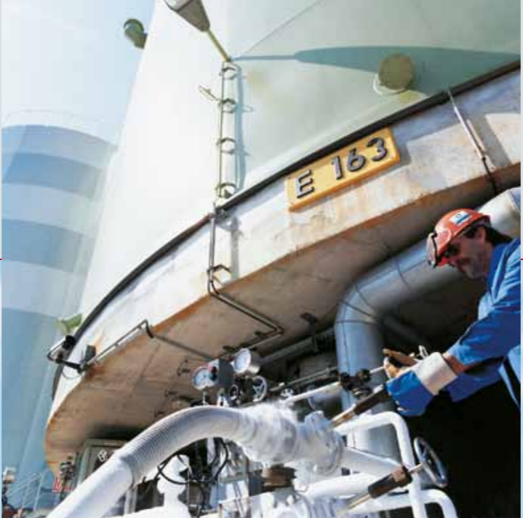
Self-operated regulators maintain the right pressure
